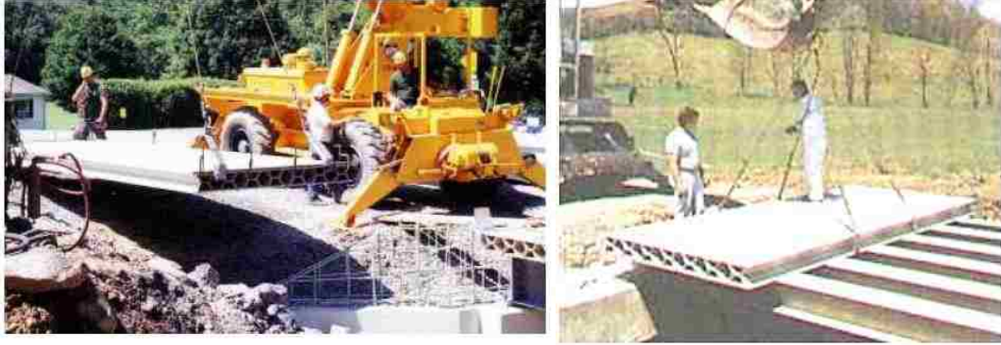
Figure 2.4. The Wickwire Run Bridge in Taylor Co., WV
